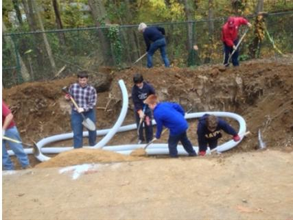
of perforated pipe at the bottom of the 5 foot deep trench to form an underdrain. The underdrain pipe outflow was positioned about 18 inches above the bottom of the trench, enabling a retention basin of the same depth.
